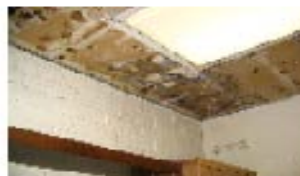
Interior wall failure Water infiltration—ceiling Slab failure throughout
